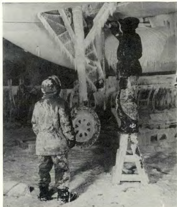
Above, the armament of an F-101 is cold weather tested. Right, an ice-crusted B-47 outrigger gear is cold soaked.
