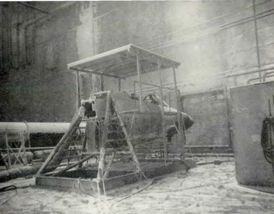
Above, the armament of an F-101 is cold weather tested. Right, an ice-crusted B-47 outrigger gear is cold soaked.
